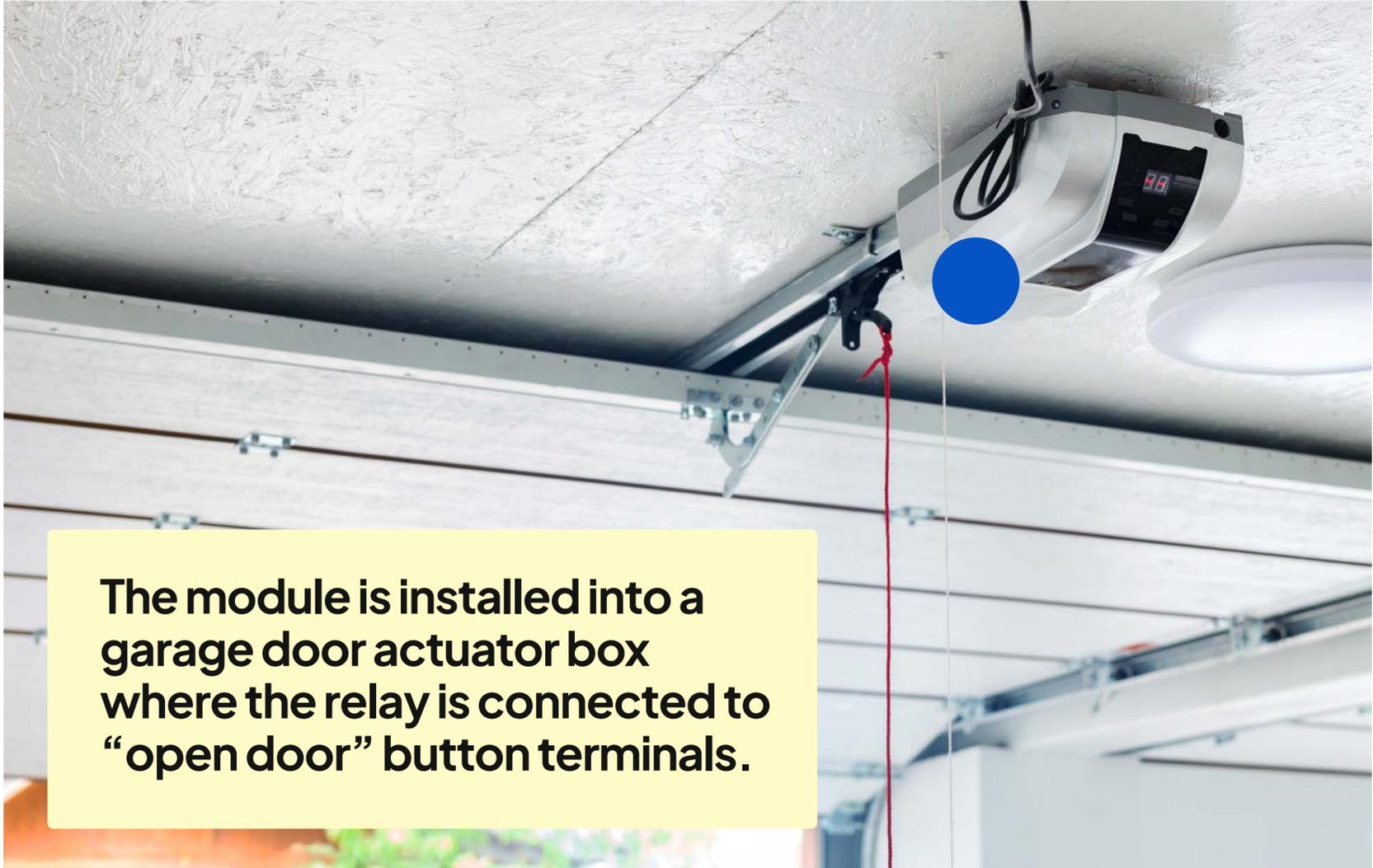
The module is installed into a garage door actuator box where the relay is connected to “open door” button terminals.
